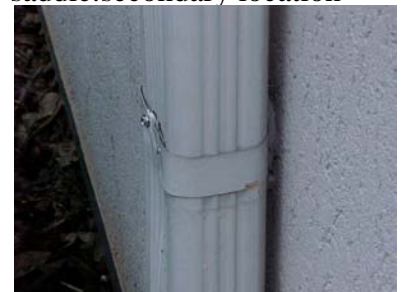
Caulk downspout attachments
