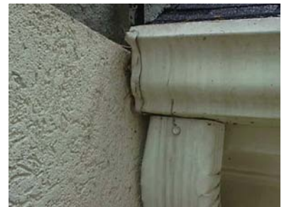
Gutter below kickout
