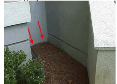
Small area foam in ground contact
