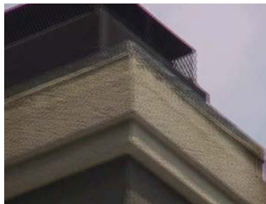
Chimney cap covers entire top of chimney
