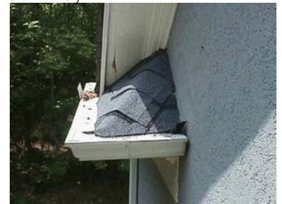
Kickout installed at roof saddle:secondary location
