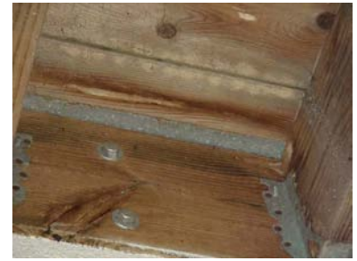
Deck flashing installed
