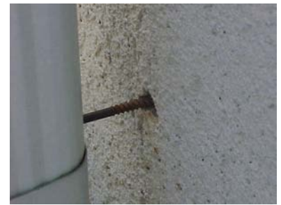
Downspout connection hole
