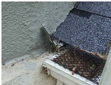
Kickout installed
