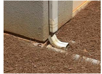
A-8: Repair downspout
