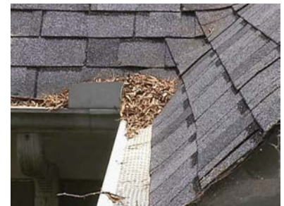
B-3: Clear leaves from gutter/roof
