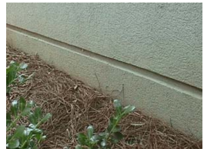
Termite band is installed
