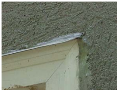
Flashing at garage
