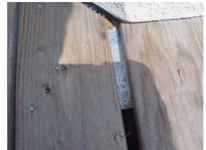
Deck flashing installed
