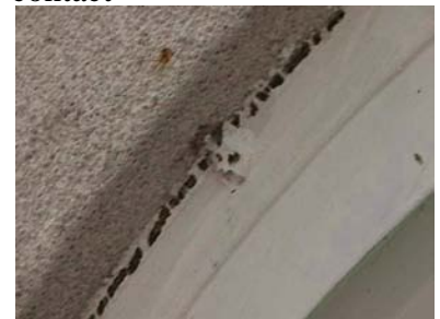
D-3: Need to caulk at half round window
