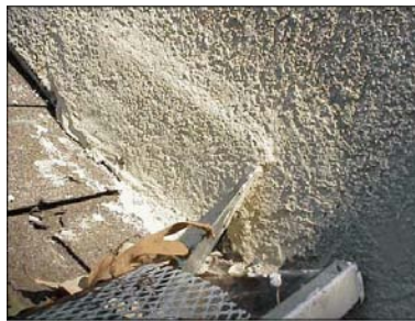
D-2: Kickout caulked to shingle
